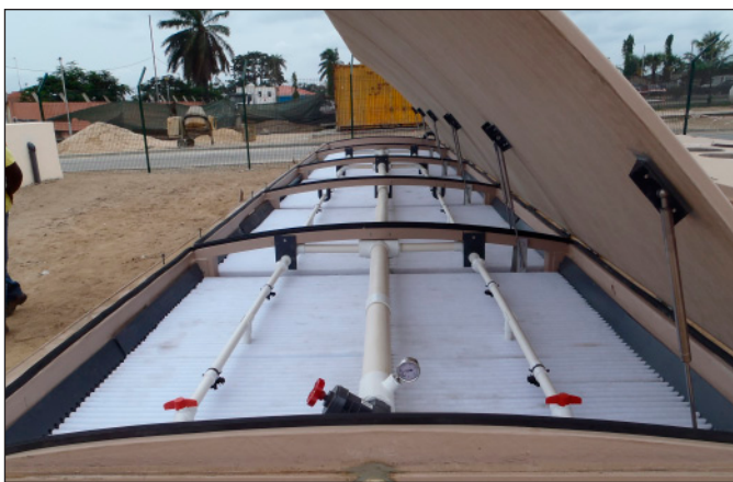
One of the 35' long (10.7 m) AX-Max units is filled entirely with engineered textile filter media. A manifold with spray nozzles disperses the effluent evenly over the textile, to optimize treatment.
