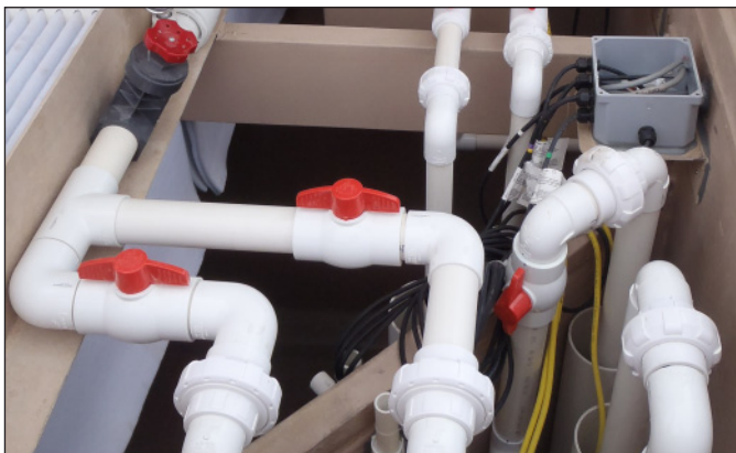
One end of the second AX-Max unit holds all the pumping and electrical equipment for the treatment system in a compact space that is easy to access for installation, operation, and maintenance.
