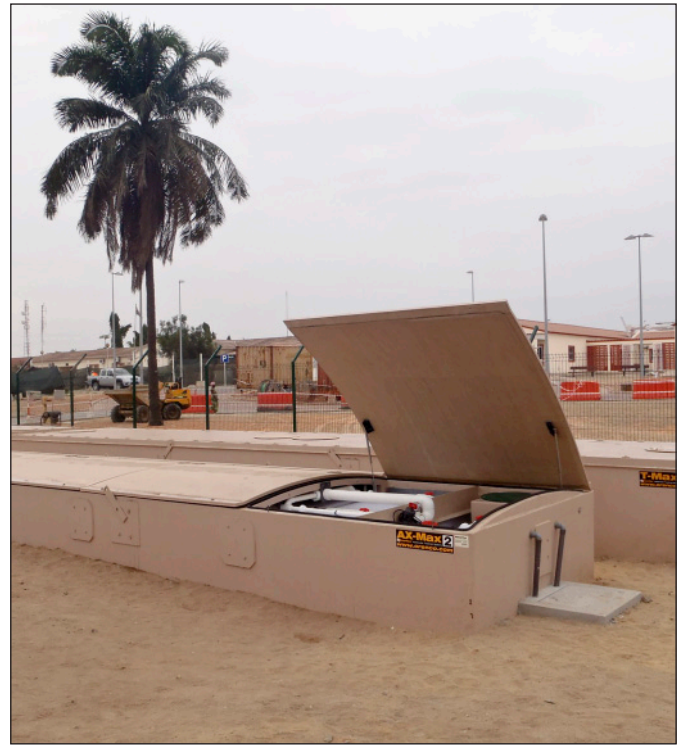
Seven-foot-wide (two-meter) lids with hydraulic shocks allow operators to quickly inspect and maintain the AX-Max filter units. Lids are then re-secured for safety.
