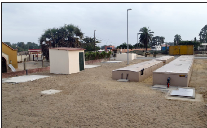
Wastewater from the hospital gravity-flows to a lift station (wet well) seen at bottom right. From there it's pumped to the two T-Max tanks for primary treatment followed by the two AX-Max filter units, where it is recirculated an average of four times before being pumped through the UV unit housed in the small controls building shown at left. Following UV disinfection, the final effluent is conveyed to the four infiltration wells surrounding the controls building, for subsurface dispersal.
