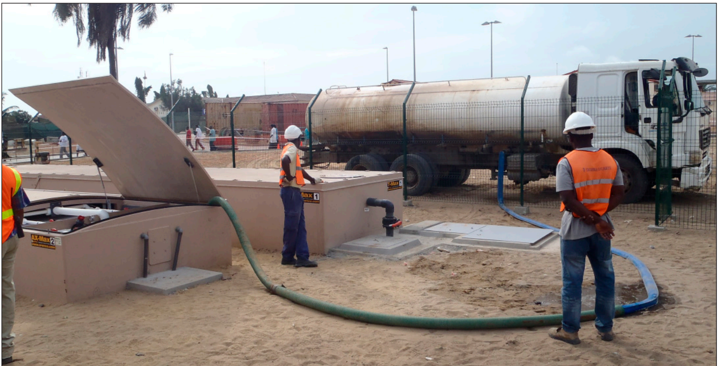
Seven-foot-wide (two-meter) lids with hydraulic shocks allow operators to quickly inspect and maintain the AX-Max filter units. Lids are then re-secured for safety.
