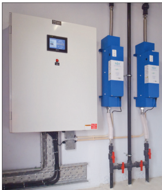
The Orenco® TCOM™ control panel includes a touch screen programmed in both English and Angolan Portuguese. Two UV Pure Hallett™ 30 disinfection units are also housed in the secure controls building at the site.
