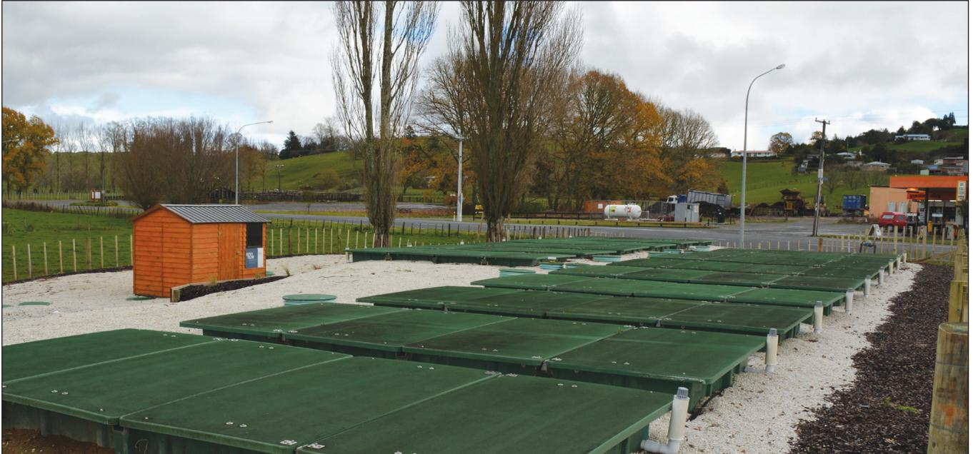
Located on the edge of the township, the fifteen AX-100 units at Piopio's wastewater treatment plant draw little attention, as they are low-profile and emit no sounds or smells. These low maintenance units can also be installed further above ground, if desired.
