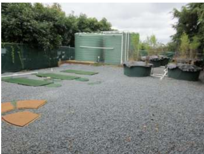
An Orenco AX60 textile filter, multiple-barrier disinfection process and captive dispersal system has replaced the failing sand filter at Gallery Walk
