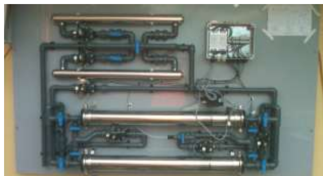
A 4-stage disinfection process has been developed at Gallery Walk for Class A+ reuse
