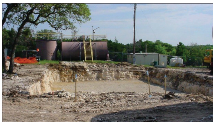
Sitework for the new, low-profile wastewater treatment plant at Morgan's Point Resort. Its rusting activated sludge plant can be seen at the rear.
