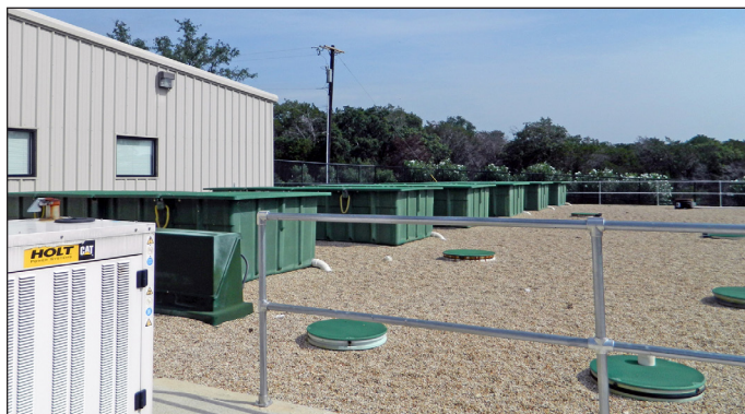
Six AX-100 pods provide all the treatment capacity the city currently needs, plus room to grow. These low-maintenance units can be installed in-ground or partially bermed, for an even lower profile.
