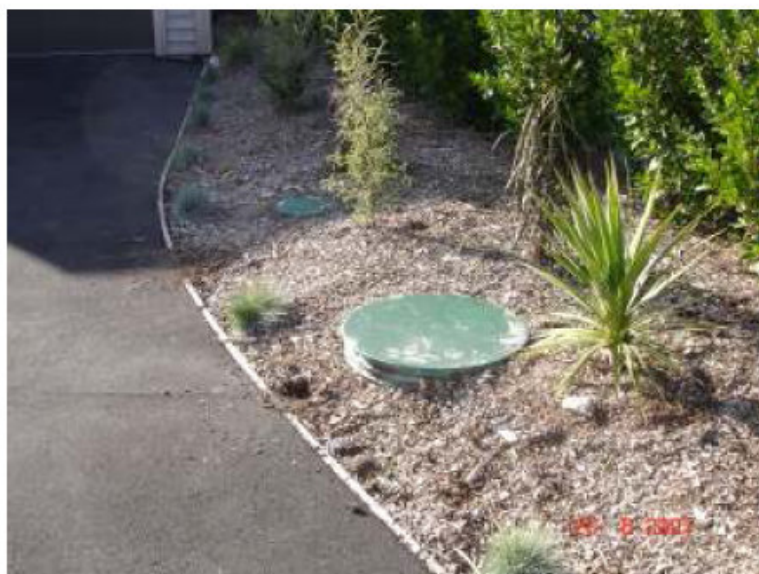
Figure 2. On lot STEP tank
