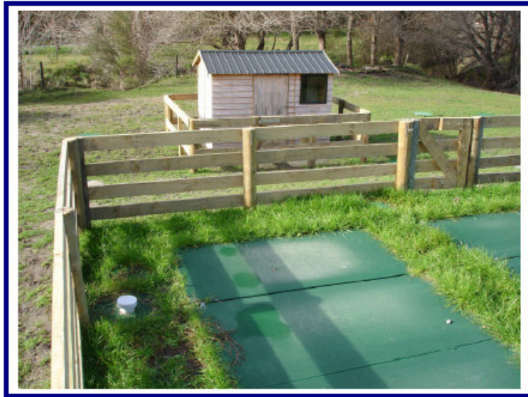
Figure 1. – AdvanTex® Treatment System and Control Shed
