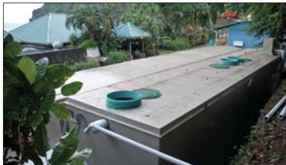
The AX-Mobile comes as a complete, fully-plumbed package. The fiberglass tanks are lighter than concrete and, at only 8' wide, these were easily trucked to the site, down steep narrow roads, on the back of a flatbed.
