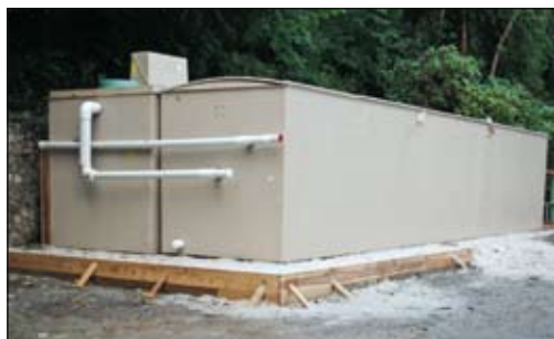
The resort needed two AX-Mobile units — one for tankage and one for treatment — to meet its emergency wastewater needs. These two units will become part of the resort's permanent wastewater solution, after equipment from the ruined system is removed.
