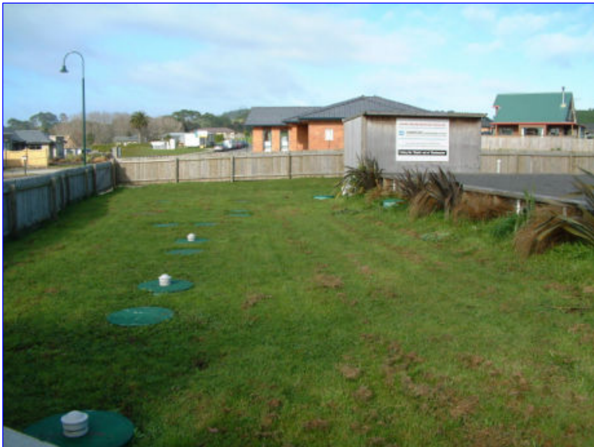
Figure 2. Photo showing the rPBR treatment system bed and tanks area.
