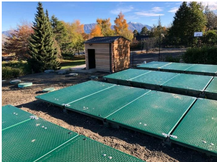
Figure 1- AdvanTex wastewater treatment plant that services the existing Lakeside Estate subdivision
