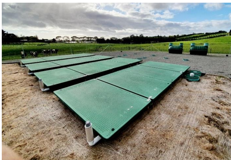
Figure 7-Photo of AdvanTex wastewater treatment plant installed to service the Ongare Point community
