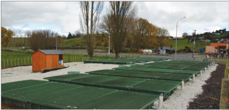
Figure 16-Photo of AdvanTex wastewater treatment plant at Piopio Community
