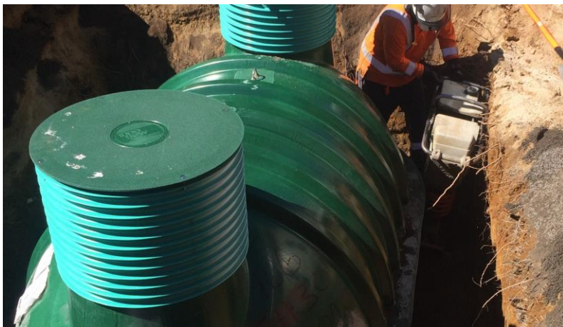
Figure 19-Photo of on-lot tank being installed
