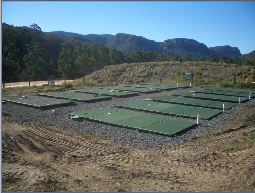
Figure 2. The AdvanTex Treatment system following backfilling
