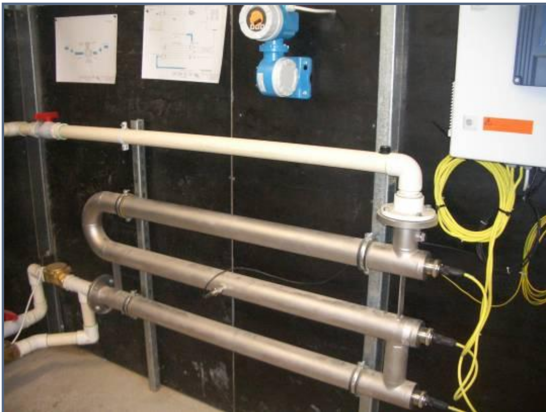
Prominent's Dulcodes 'D' UV system provides stage-1 disinfection to the effluent before storage in the Irrigation Supply tank
