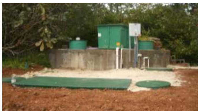
Orenco's AdvanTex® Recirculating Textile Filter, coupled with the existing tank onsite provides a robust solution for the cheese processing waste
