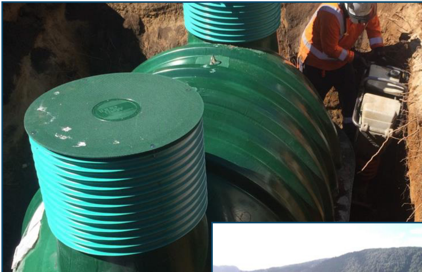
Figure 19-Photo of on-lot tank being installed
