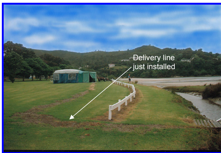
Figure 3. The delivery line was small bore polyethylene.
