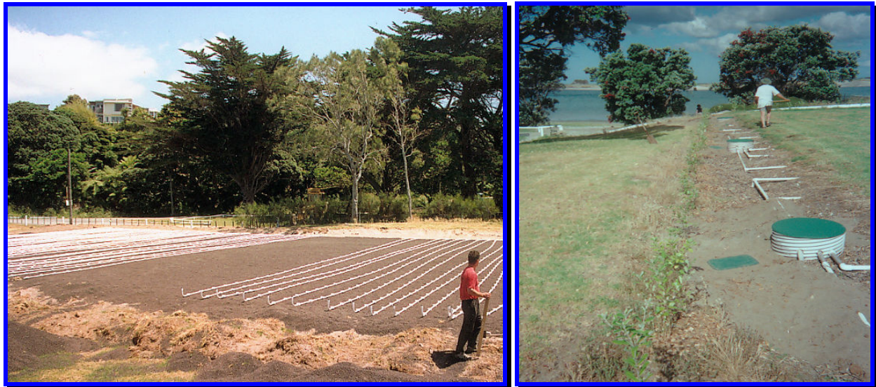
Figure 4. The distribution system and sequencing valve layout.
