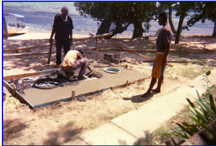
Figure 3. Installing the tanks.
