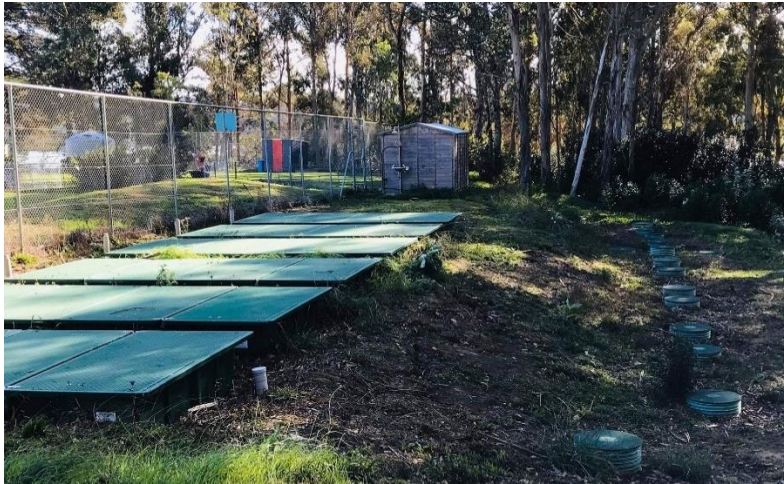
Waiheke School's AdvanTex® Wastewater Treatment System
