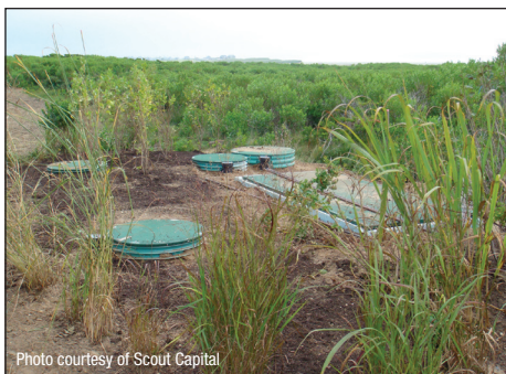
An AdvanTex® Treatment System, manufactured by Orenco, nestles discreetly in the beach grass. This low-energy, highly reliable media filter replaced the former cesspool and treats this Esther's Island household's wastewater to re-use quality.
