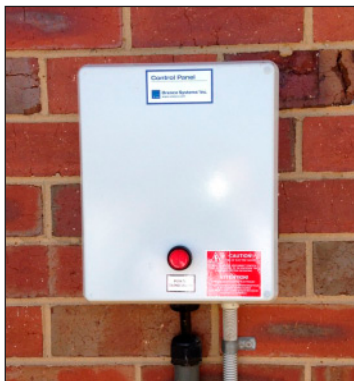
A programmable control panel at each home monitors the components of the on-lot STEP package.
