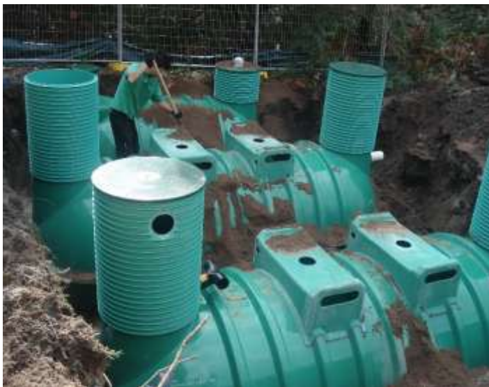
The InnoFlow/Orenco fibreglass primary and recirculation tanks being installed in June 2010 by Kerry Flanagan Wastewater
