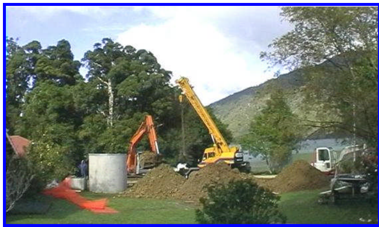
Figure 3. Installing the tanks.
