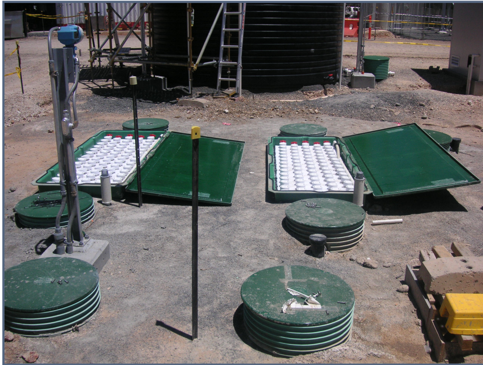
Two of Orenco's AX20FAPs, approved in Queensland for residential use, operate in parallel to treat all domestic wastewater onsite
