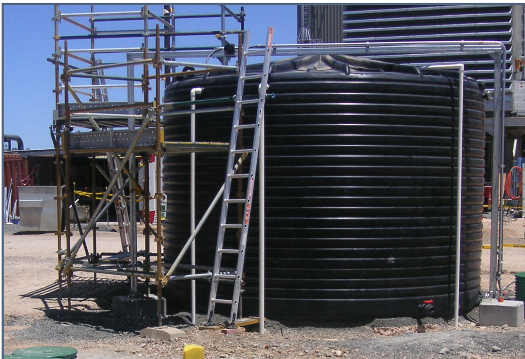
To allow for use of the recycled water when it is needed rather than when it is produced, the system includes a 2-week above-ground storage tank
