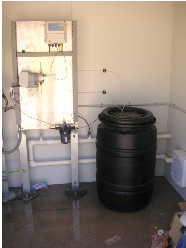
The chemical shed at the treatment plant houses the chlorine drum dosing pump, recirculation loop and main treatment plant controls
