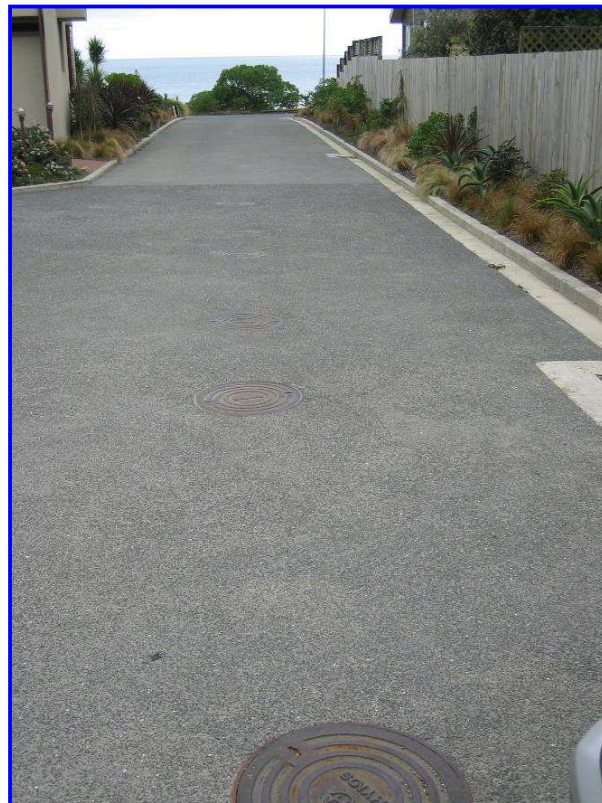
Figure 2. A low visual impact was important for this installation. Trafficable riser covers can be seen clearly in this photo.
