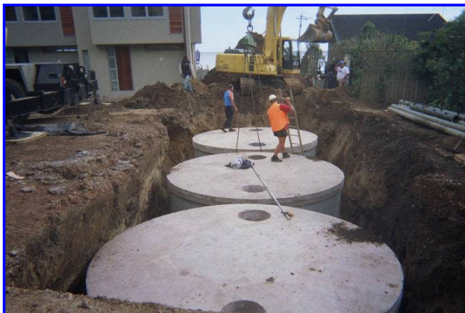
Figure 4. Installing the tanks.
