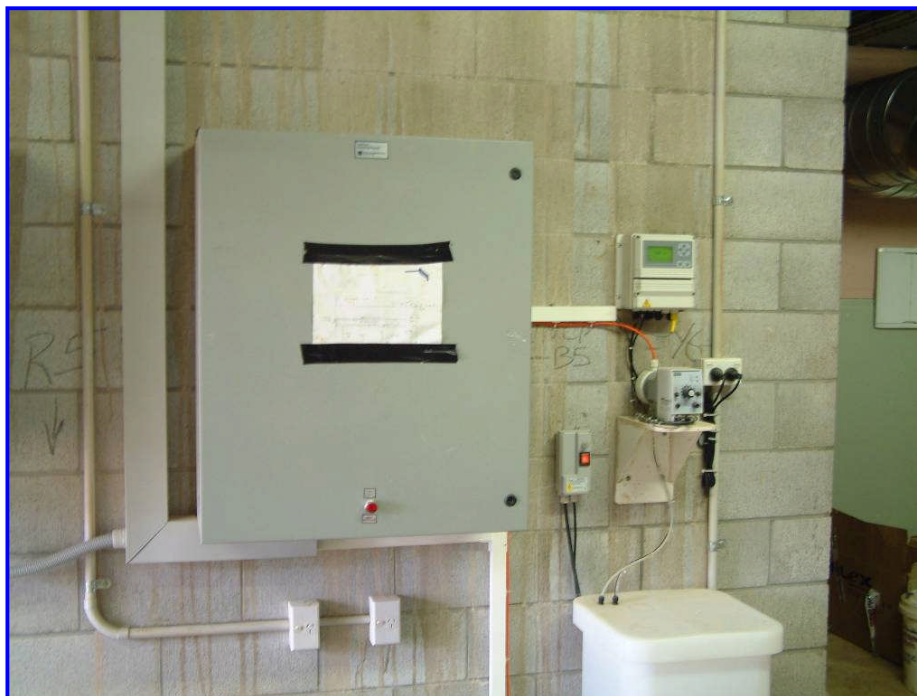
Figure 6. Control Panel and RTU
