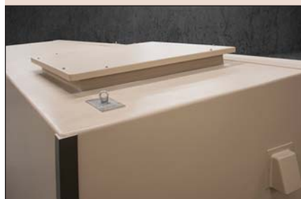
The two-room water utility building houses the water system’s booster pumps. It has a custom hatch on the roof to allow for easier pump removal.
